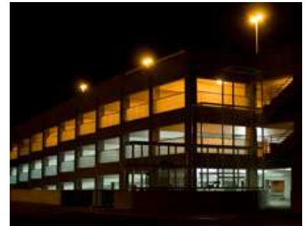
Street view shows evident color difference halfway into installation
