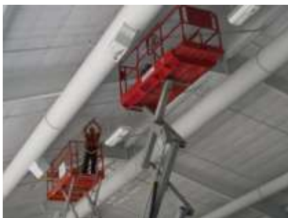
Installation of EverLast® 400w High Bays
